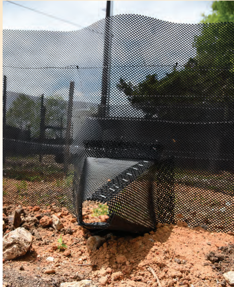
To be effective, toad exclusion fences need to prevent climbing and have jumpouts (pictured above) to allow toads to escape construction zones.
