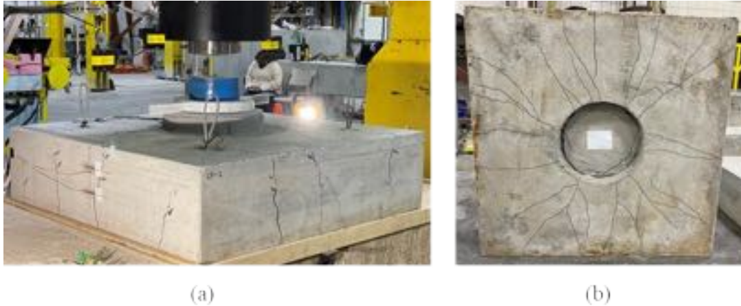
Figure B - 14: Cracking after testing on (a) south-west side and (b) bottom of the Specimen LP-2.
