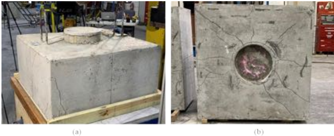
Figure A - 35: Cracking on (a) cap and (b) bottom of the Specimen S2-3
