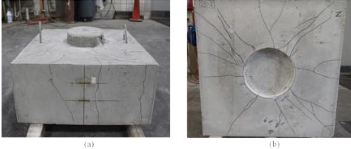
Figure A - 127: Cracking after testing on (a) east side of cap and (b) bottom of Specimen S3-2.
