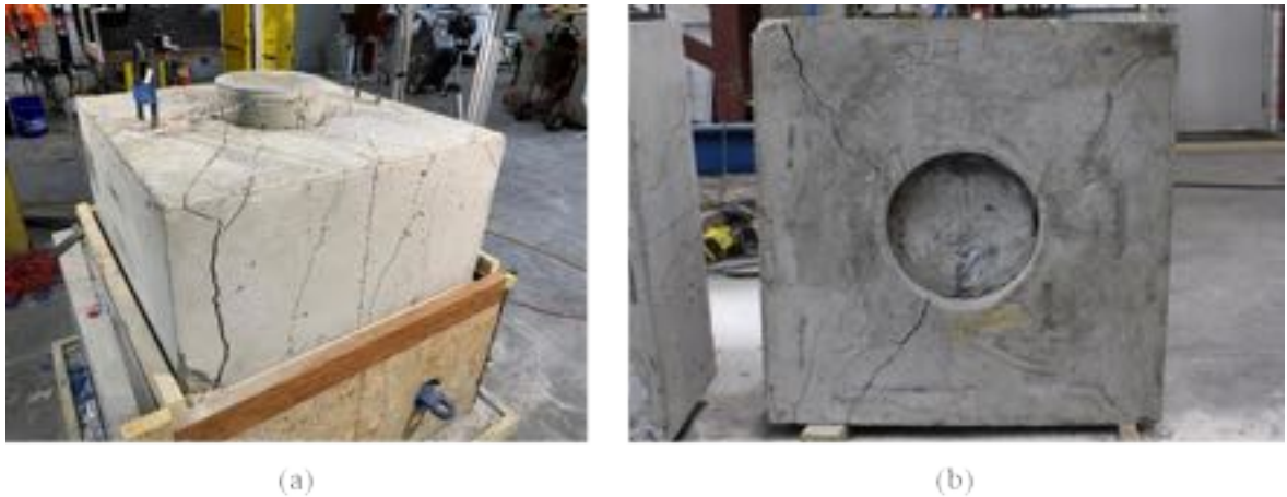
Figure A - 59: Cracking on (a) cap and (b) bottom of Specimen S2-7
