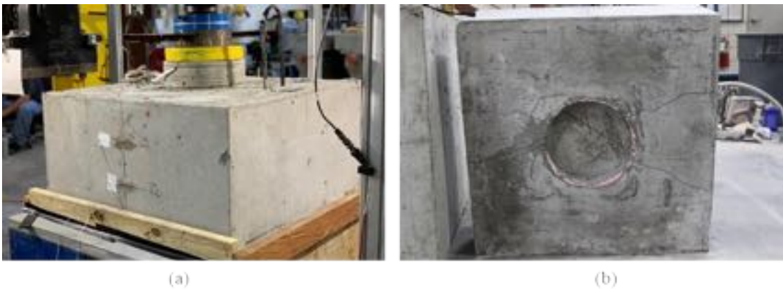
Figure A - 29: Cracking on the (a) surface of the cap and (b) bottom of the specimen S2-2
