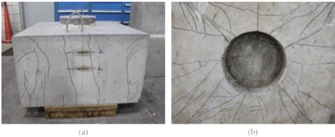
Figure A - 97: Cracking on the (a) east side and (b) bottom of specimen S2-13
