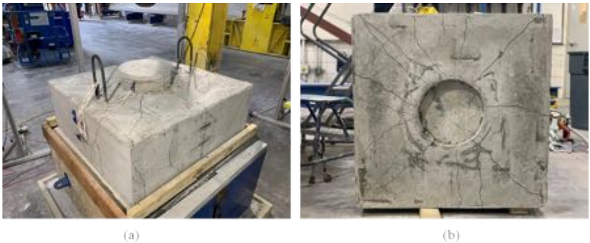
Figure A - 47: Cracking on a (a) cap and (b) bottom of the Specimen S2-5
