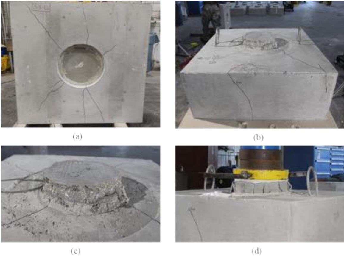
Figure A - 191: Failure details on (a) bottom, (b) cap, (c) top of plug and (d) plug detail during testing of the Specimen S3-13
