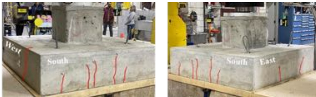
Figure B - 45: Crack pattern at 350 kips for SC-1
