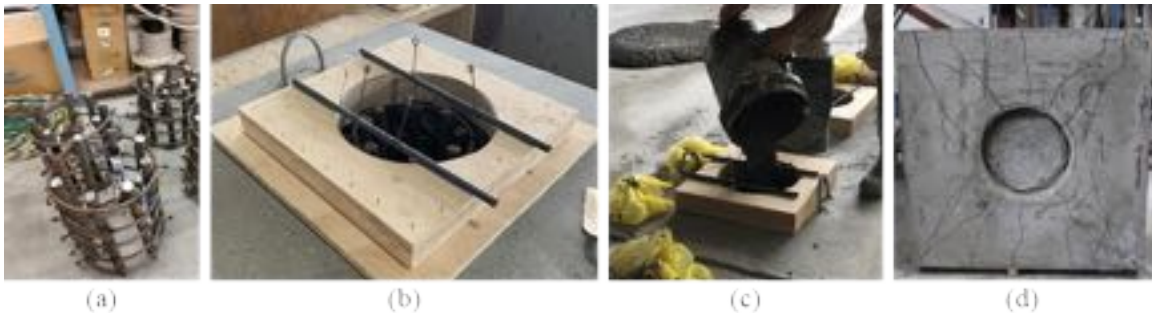
Figure 3-4: Plug construction: (a) typical plug reinforcement, (b) 3-inch cylindrical form on top of cap, (c) casting of plug concrete, and (d) 3-inch blockout on bottom of plug (after testing)
