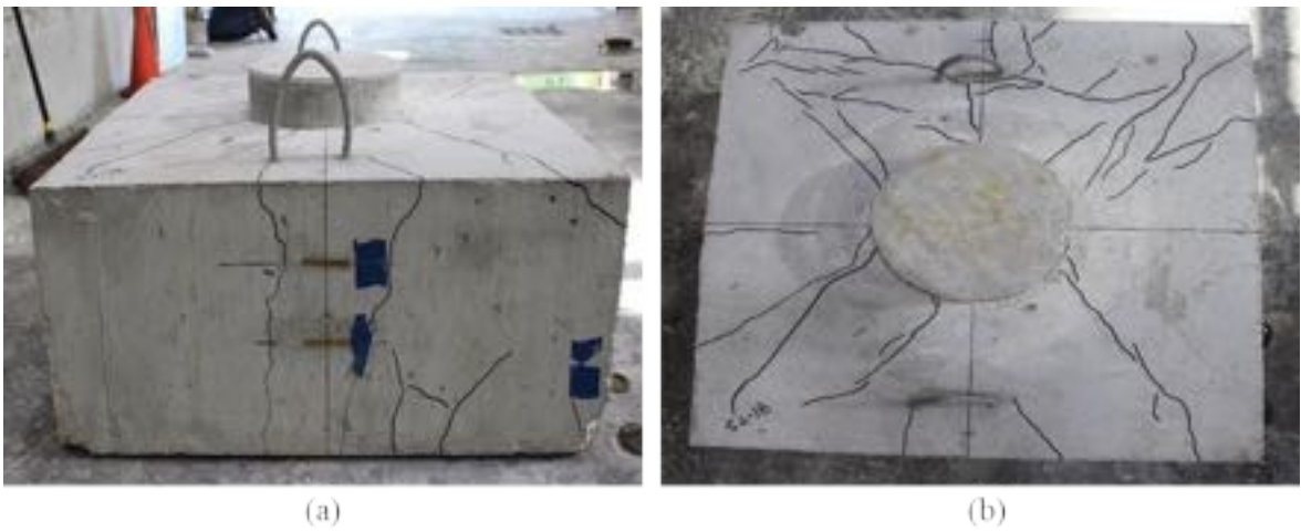
Figure A - 112: Cracking on the (a) east side and (b) top of the specimen S2-18
