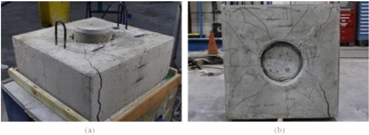
Figure A - 84: Cracking on (a) cap and (b) bottom of Specimen S2-11
