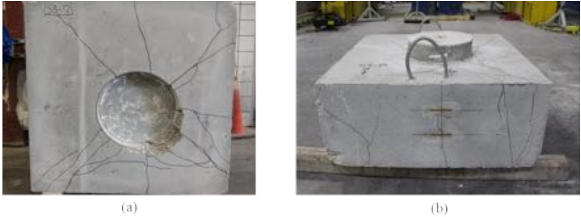
Figure A - 185: Cracking after testing on (a) bottom and (b) cap of Specimen S3-12
