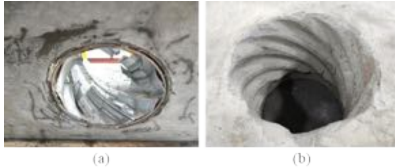
Figure 3-3: (a) Removal of corrugated pipe and (b) surface finish after removal of pipe and sandblasting
