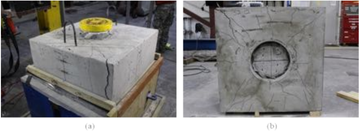
Figure A - 90: Cracking on (a) cap and (b) bottom of Specimen S2-12
