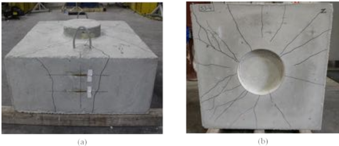
Figure A - 138: Cracking on (a) cap and (b) bottom of Specimen S3-4
