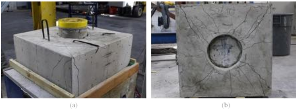
Figure A - 78: Cracking on (a) cap and (b) bottom of Specimen S2-10
