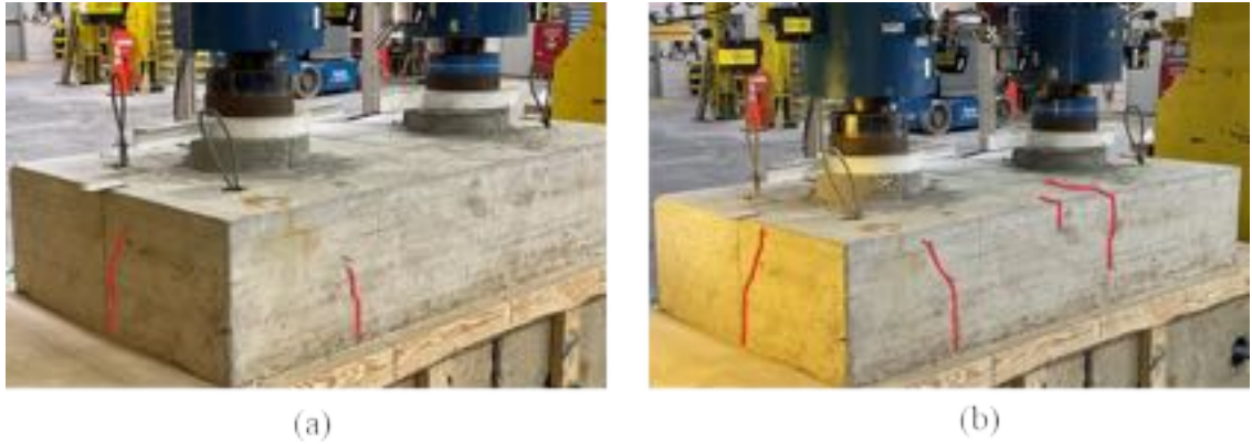
Figure B - 32: Crack propagation during testing at (a) 150 kips and (b) 250 kips on MP-1 Total load on the system (i.e., both plugs) plotted versus concrete strain for MP-1 are shown in Figure B - 33. Cracking was first observed with the CSGs around 180 kips to the north of the west plug, see CSG-PCN5 and CSG-PCN6. Generally, compression strains were measured on the north face between the plugs and toward the east side of the specimen.
