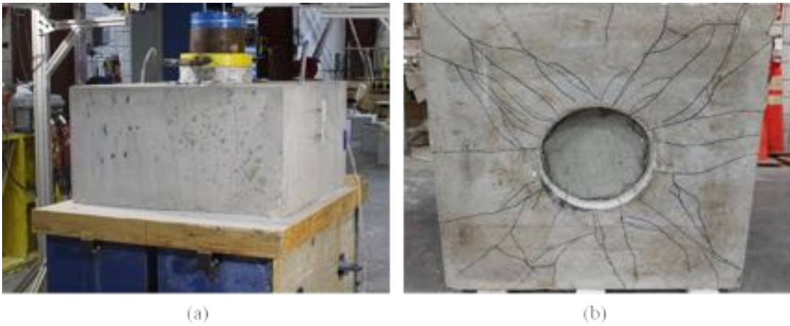
Figure A - 118: Cracking on the (a) south side and (b) bottom of the specimen
