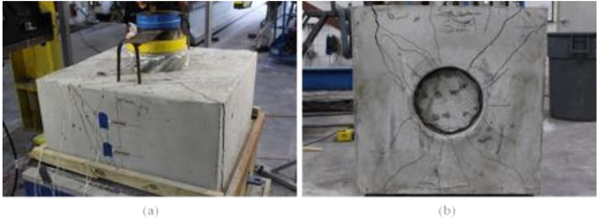
Figure A - 71: Cracking on (a) cap and (b) bottom of Specimen S2-9
