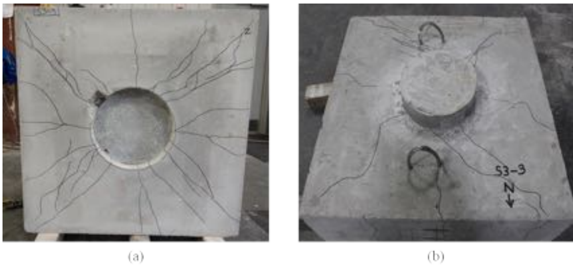
Figure A - 132: Cracking after testing on (a) bottom of the cap and (b) top of the cap of Specimen S3-3
