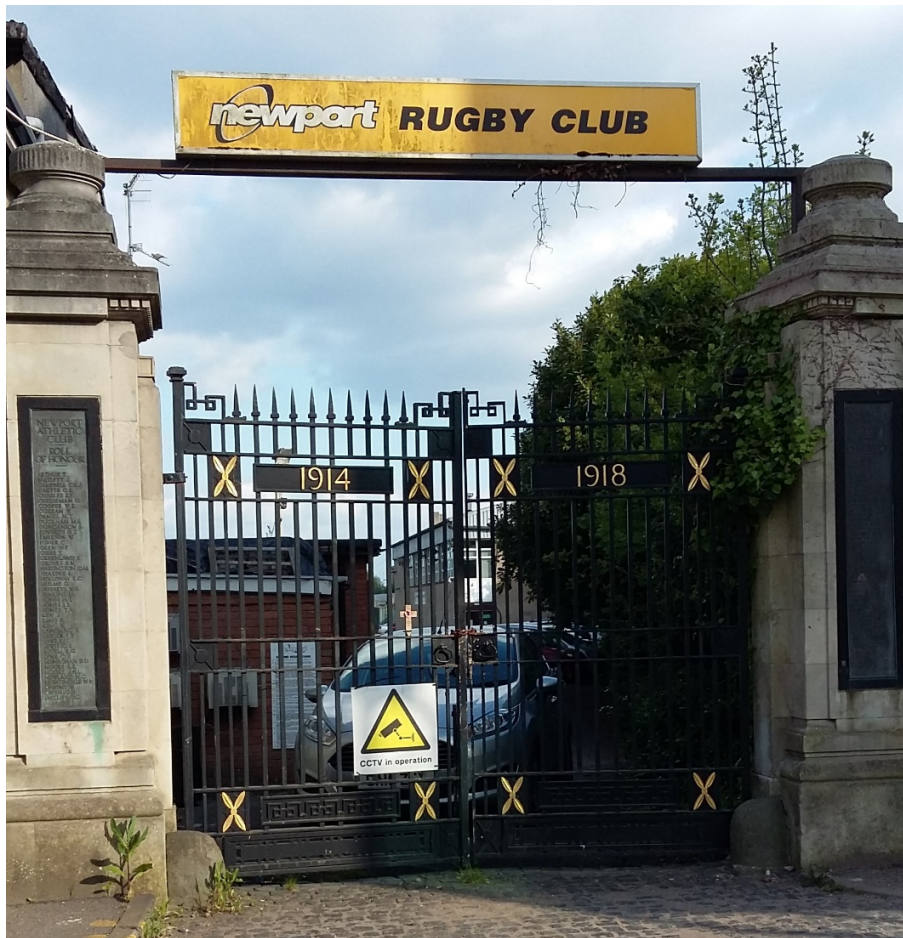
Fig. 16 Memorial Gates, Rodney Parade. Unveiled by Lord Tredegar September 6 1923. Eightyfive Service members of Newport Athletic Club are listed on the column tablets as a Roll of Honour, not as being lost in action. The Gates were until recent times the main public entrance but have since fallen into disuse and neglect. Rodney Parade now hosts two rugby teams and Newport County AFC. Examination of the names listed shows very few directly Welsh surnames and perhaps comments on the overall composition of the Club itself. There is little reference to the details of death, one name that is mentioned is 'Phillips, L.A.' listed as a Sergeant in the London Royal Fusiliers, killed at Cambrai, March 14, 1916. https://www.iwm.org.uk/memorials/name/466784 .
