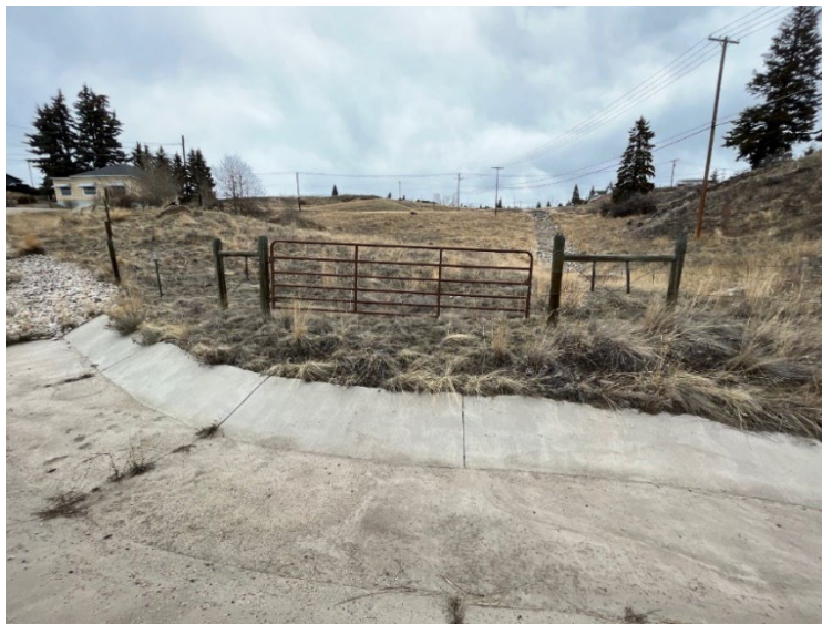
Photograph 7: Overview of Buffalo Ditch looking north.
