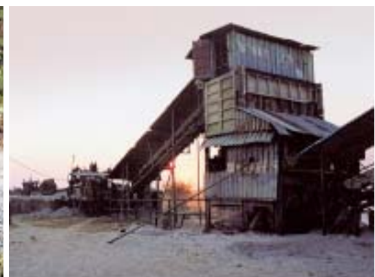
Lilyvale Farm lime plant, Zambia.
