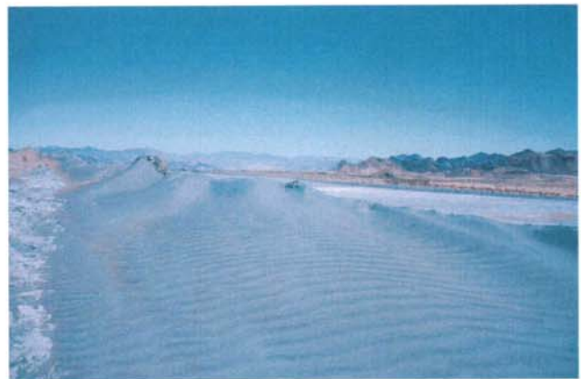
Dunes formed from fine tailings on top of heap as a result of reworking by wind.
