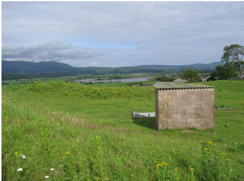
Figure 9 Typical shed housing for borehole used for rural farm supply
