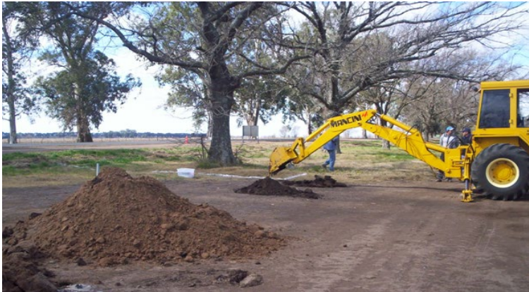
Picture 9. Soil removal tasks to monitor soil contaminated with hydrocarbons in a rural area and then remedied by stabilization methodologies (Alejo Ledesma, Argentina).
