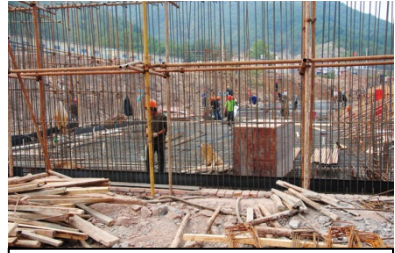
Construction site by migrant workers
