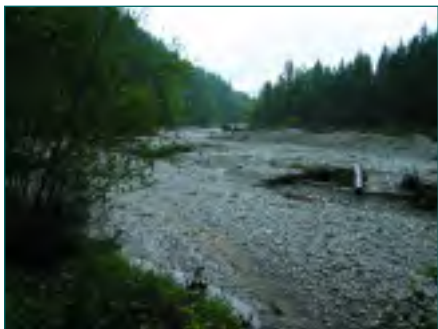
Gravel removal, upstream from ALP-7.
