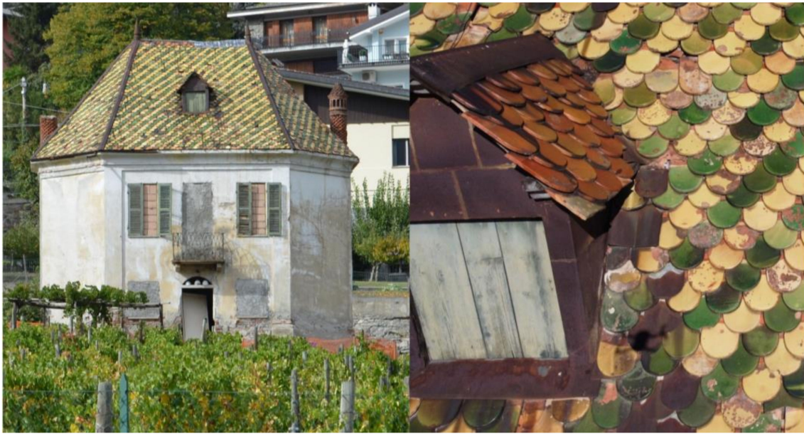
Figure 1. (Left): the 18th century pavillon “Casa delle Vigne” in Aosta (northeast Italy) with its peculiar tiles roof. (Right): the fish-scale pattern commonly used for tile alignment in roofing.
