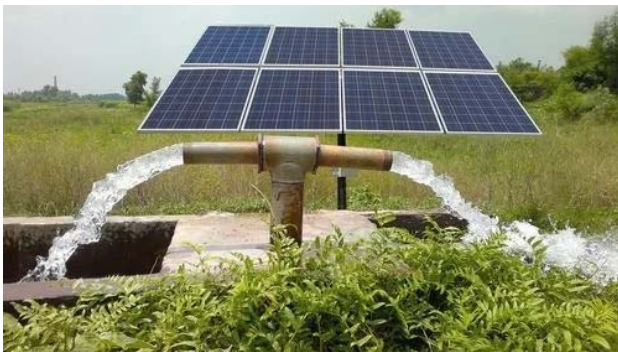
Fig. 6. Water pumping application for irrigation.
