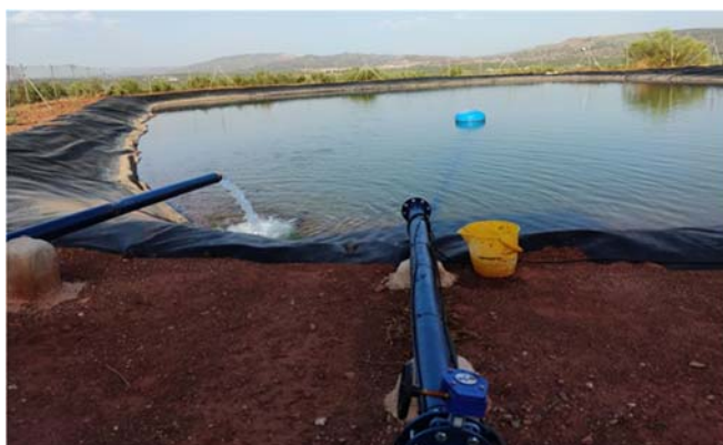
Fig. 2. Irrigation pond associated with a stand-alone photovoltaic solar water pumping installation.
