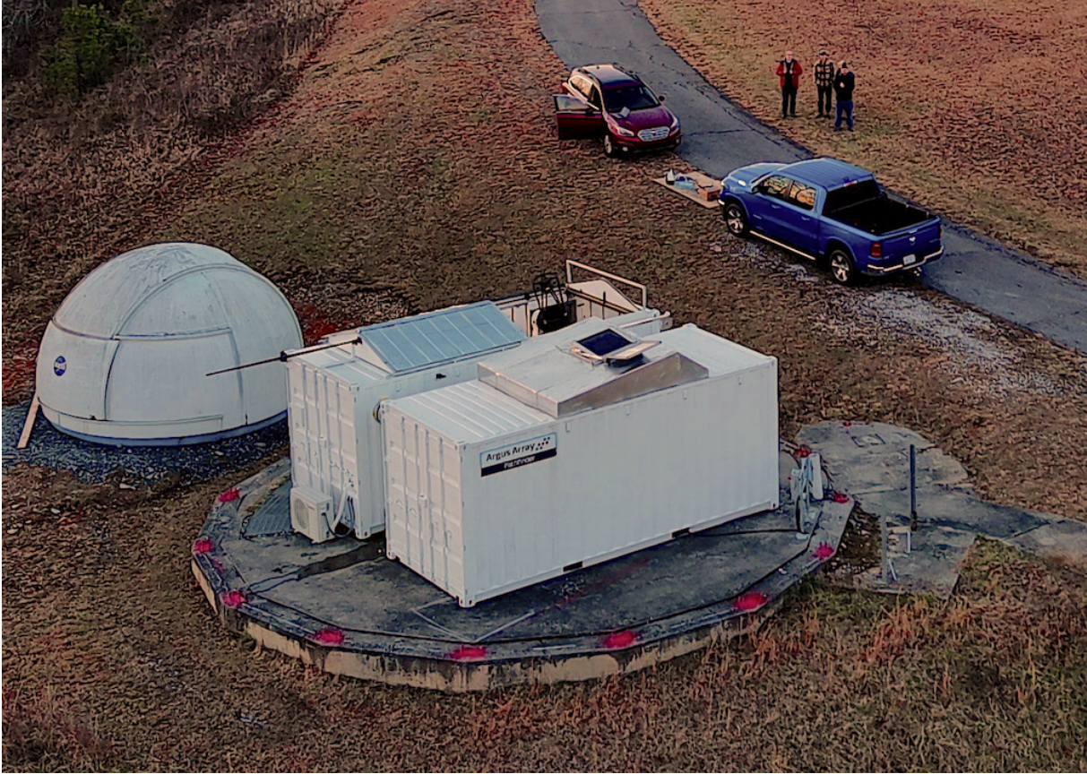
Figure 1.5 Argus Pathfinder installed at the Pisgah Astronomical Research Institute in Rosman, NC (front container). The second shipping container houses ArgusSpec (Galliher et al. 2022b), a dedicated spectroscopic followup system, and a “service module” with computing and climate control equipment.
