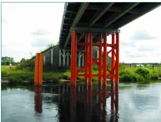
Major bridge structure on the Pisa River at PL-10.
