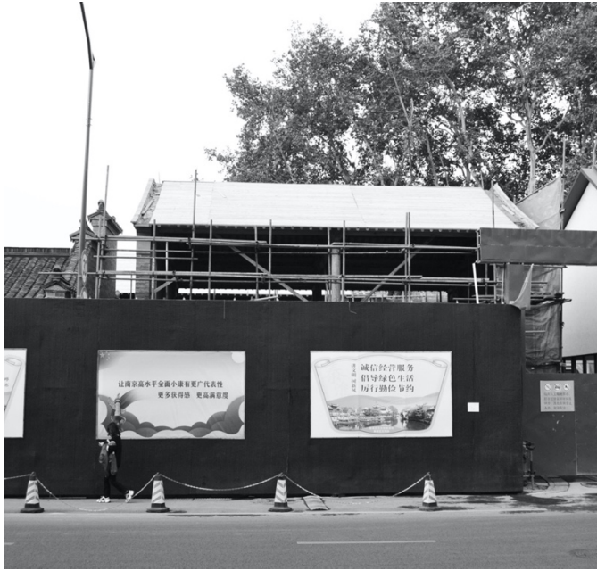
Fig. 03 - Urban regeneration works in XiaoXiHu block
