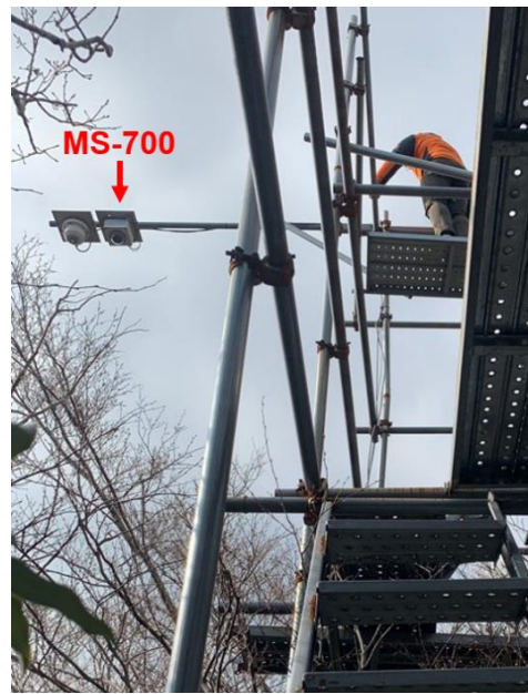
b) Installed View of MS-700 for Upwelling Irradiance Observation
