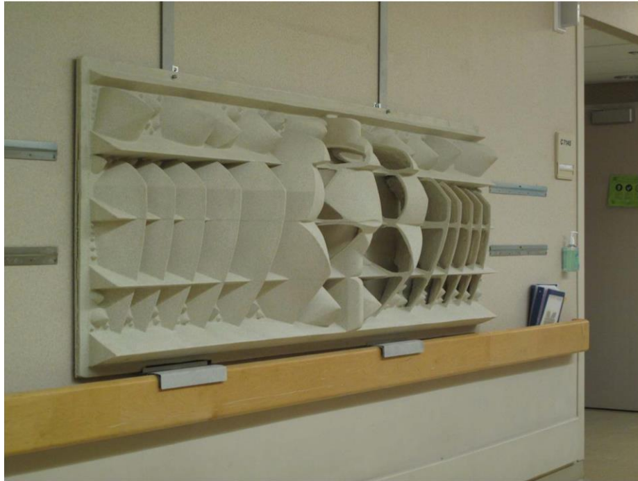
Figura 1: Panel Acústico. Fuente: Farrehi, Brahmajee y Mojtaba, 2015. This sound acoustic panel is 36×96 inches and thickness measured 3/8 inch with overall depth of 11 inches. Custom panel.
