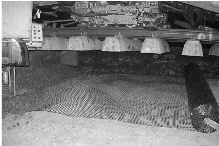
13. Laying Tensar TriAx geogrid with AHM
