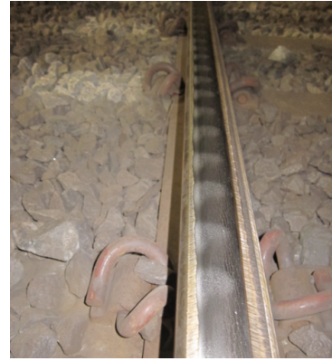
Figure 2: Example of rail corrugation from a curve in the network of Stockholm metro.
