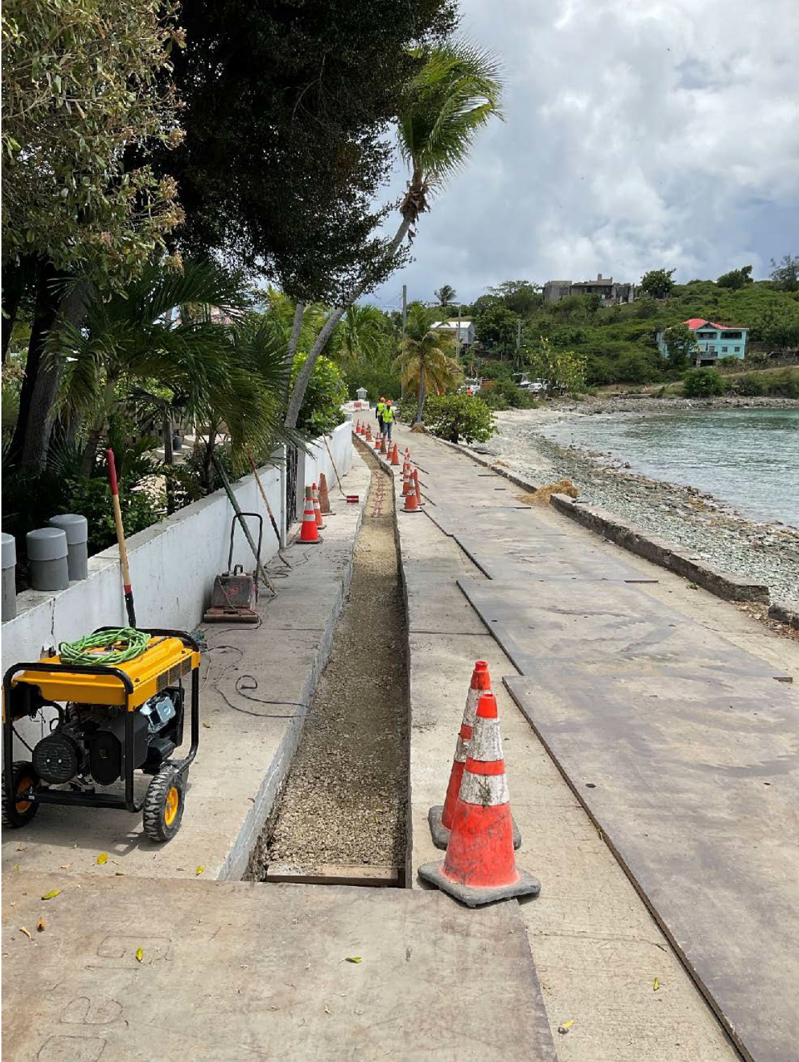
Figure 14. Installed electrical conduit along Tobacco Road, outside of the Cruz Bay Historic District, at Frank Bay. View to south.
