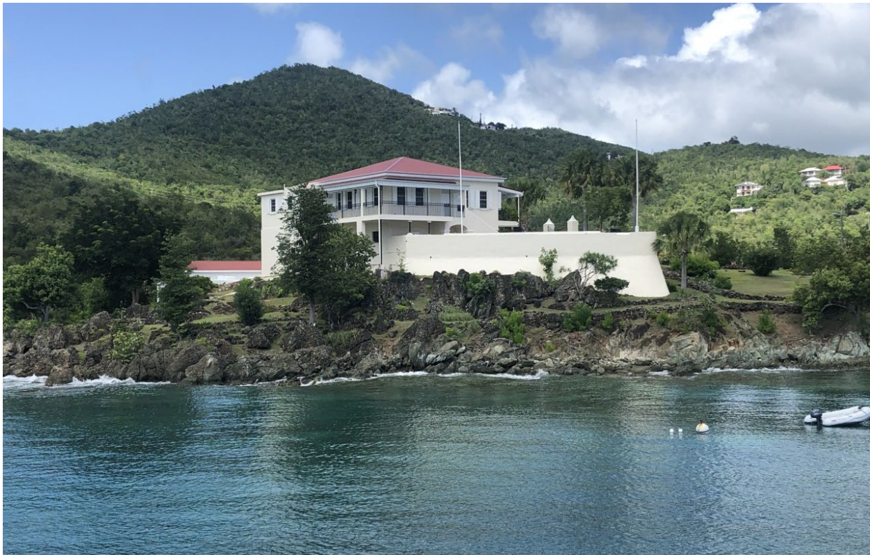
Figure 12. The Battery at Cruz Bay surrounded by steeply sloping terrain. View to northeast.
