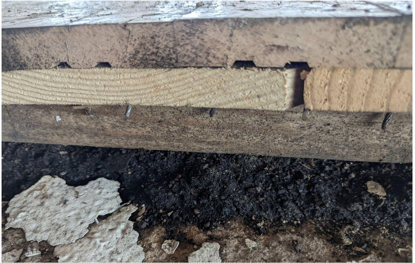
Figure 2.0 Existing Flooring (Wood, 2023)
