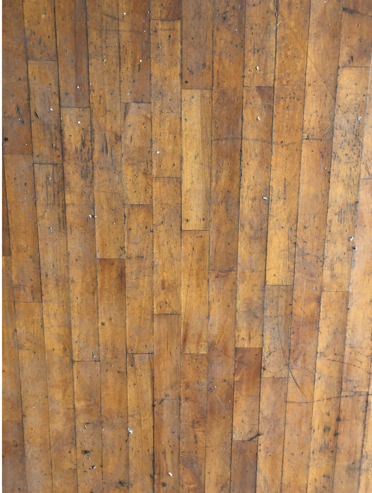
Figure 2.01 Existing Flooring (Wood, 2023)
