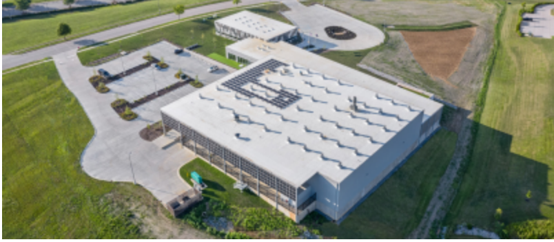
Figure 2.05 Solatube Exterior View (Solatube, 2021)
