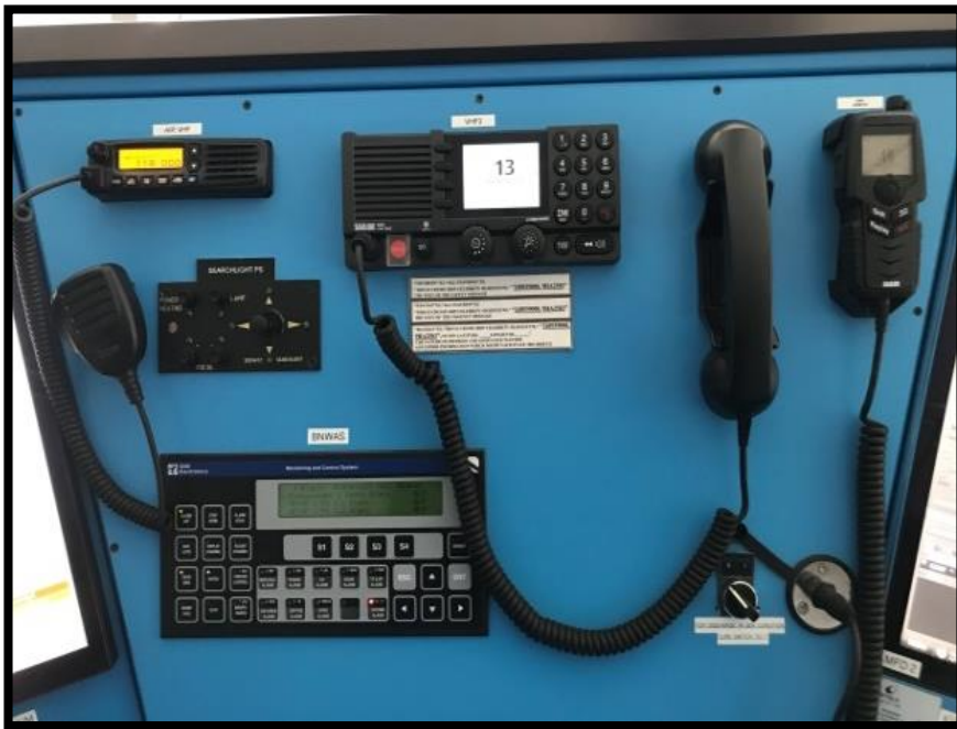
FIGURE 3-6: BRIDGE CONSOLE (SOURCE: OWN ELABORATION)
