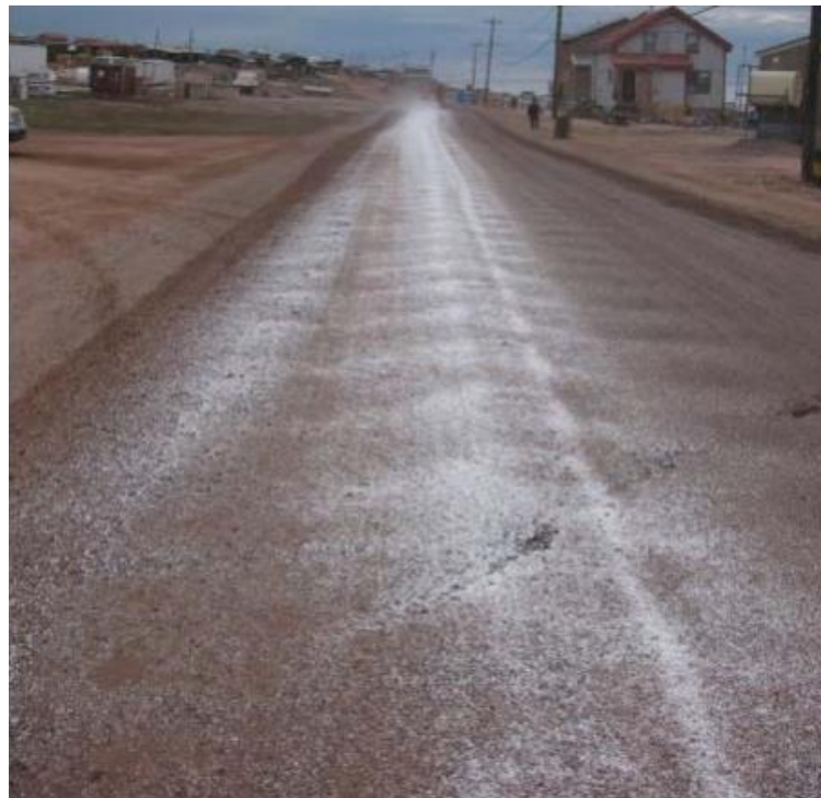
Figure 6. Road surface treated with calcium chloride.
