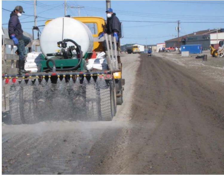
Figure 5. Applying calcium chloride uniformly across the entire width of the road.
