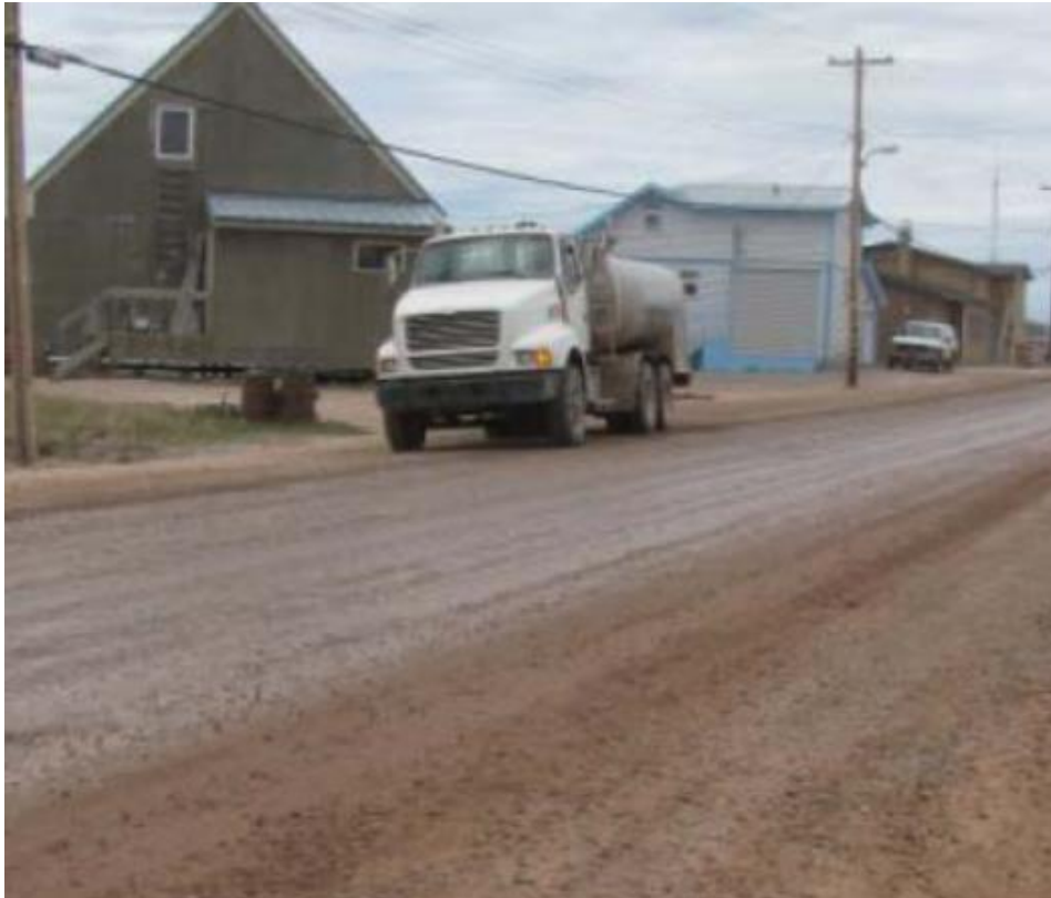
Figure 4. Watering the road surface until it is lightly saturated.
