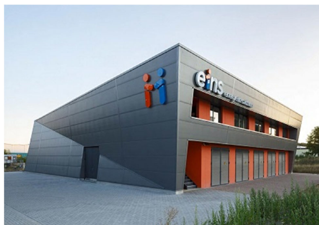
Figure 2. Image provided in urban design condition. Reproduced with permission. Copyright 2022, eins energie in Sachsen GmbH & Co. KG.
