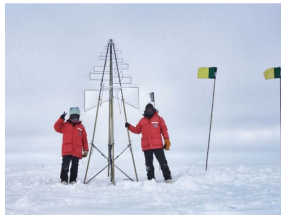
Installation of a radio antenna.
