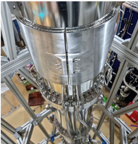
Fig. 10 Pre-cooler installed at the top of the inner cryostat vessel. LN 2 is flushed from the bottom of the outer vessel through a DN40CF liquid feedthrough up to the four-quarter circle plates, connected in series. The boil-off of the LN 2 inside the plates provides up to (0.57 \pm 0.03) kW of cooling power
