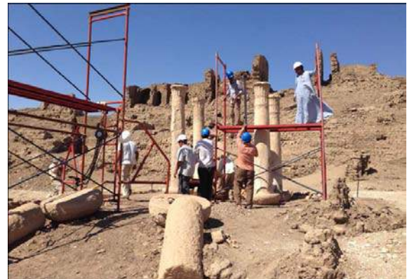
Figure 6: Site under preparation phase, scaffolding installed, 2016.
