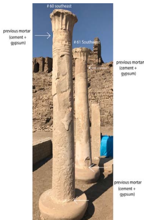
Figure 18: Shows the parts of the previous mortar used to reassemble the column of South East # 60 and the column of Southwest # 61 in 1930.
