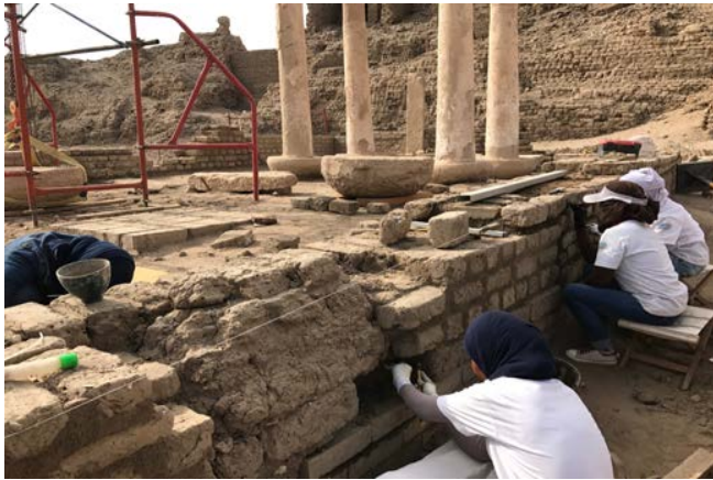
Figure 34: Replacing the damaged section with a new mud brick.
