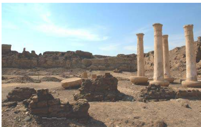
Figure 11: The conditions of the old mud brick and stone columns walls before restoration.
