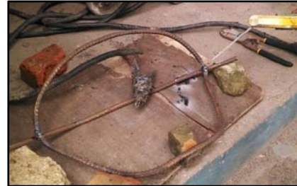
Fig. 33: Inner part of pedestal
