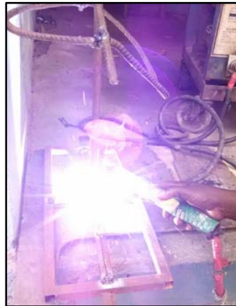
Fig. 35: welding inner to base support
