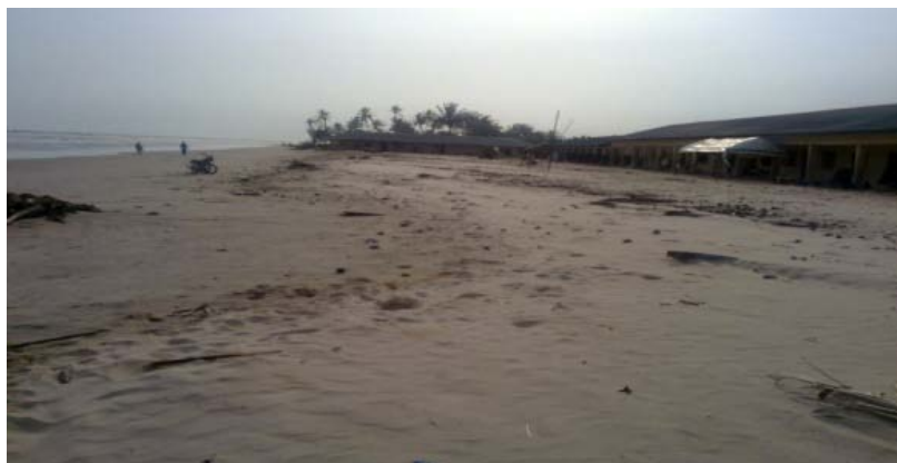
Plate 2 : Vacated School Near the Shore, Destroyed by Erosion
