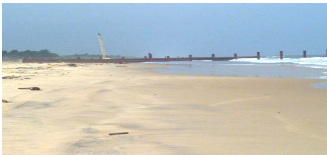
Plate 3 : Engineering Activities (Pipe-laying) on the Shore
