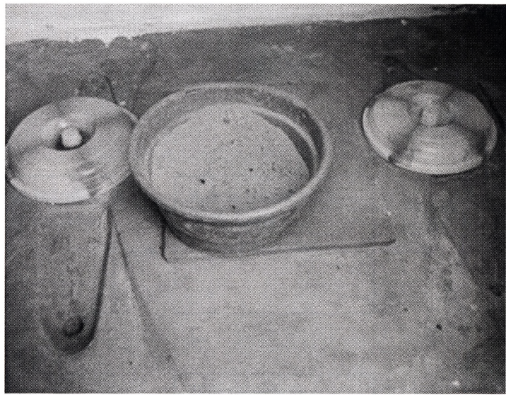
Figure 4. The floor of the EcoSan toilet. The hole covered with the lid is for the solid excreta and the hole in front is for the liquid excreta. The ash is located in the middle container. Picture taken June 2006
