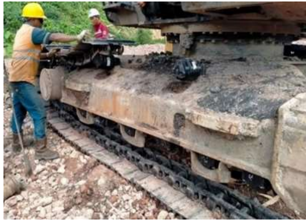
Gambar 11. Memasang Track Assembly
