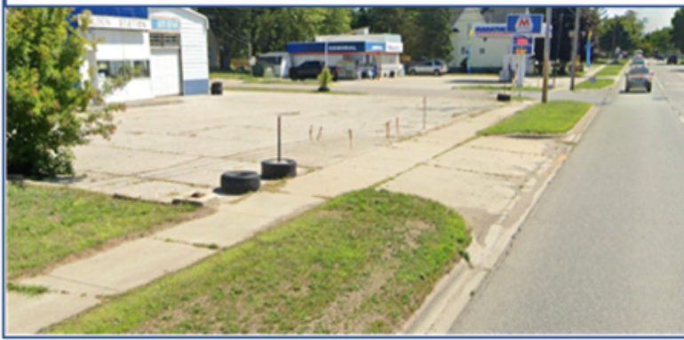
W State St: Uneven sidewalk with no ADA ramp
