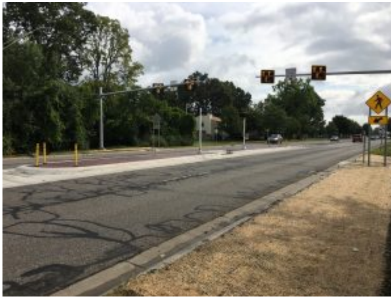
Figure 28 City of Southfield: HAWK (High-Intensity Activated Crosswalk) beacon system.
