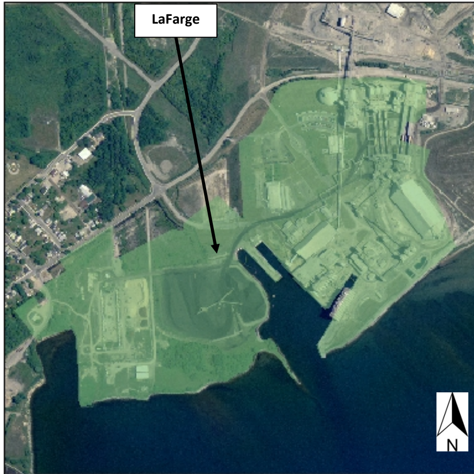
Figure 2-9 LaFarge Dock and Property
