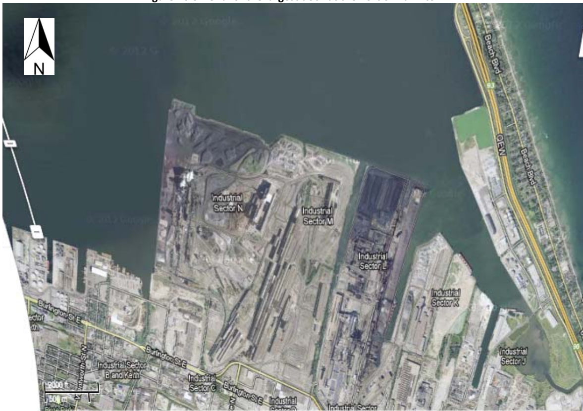
Figure 10-9 Aerial of the largest dock at the Port of Hamilton
