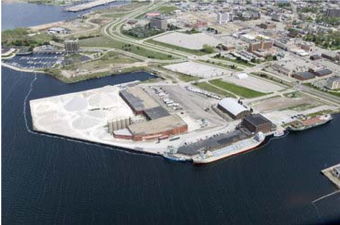
Figure 10-6 Birds eye view of the ports major loading dock and Terrace Point Marina
