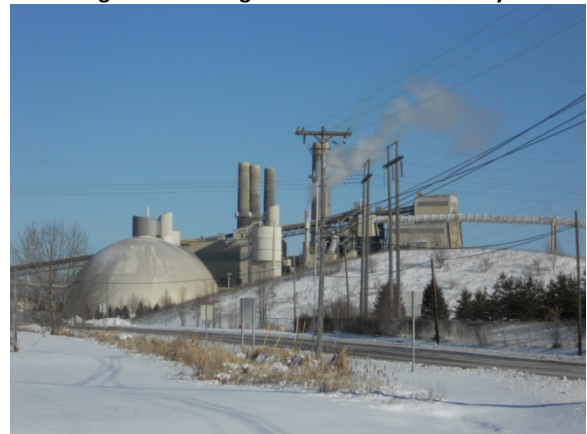
Figure 2-8 LaFarge Plant from Thunder Bay
