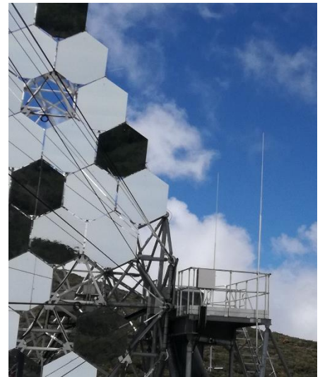
Fig. 3-21: lighting rods on the tower access
