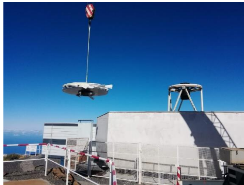
Fig. 2-51: The primary mirror suspended from the crane [76]
