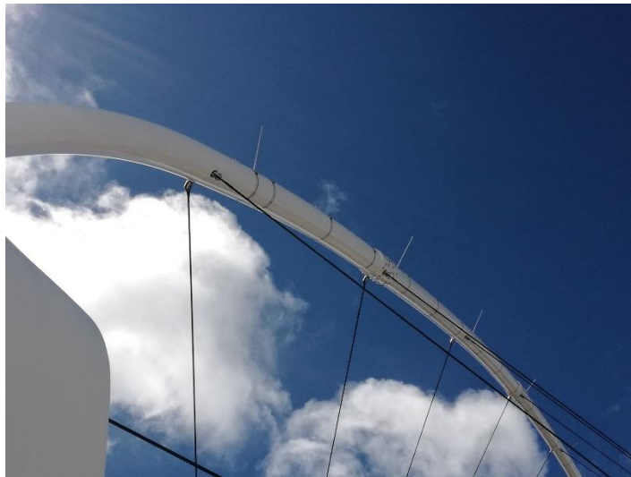
Fig. 3-20: lighting rods on the arch
