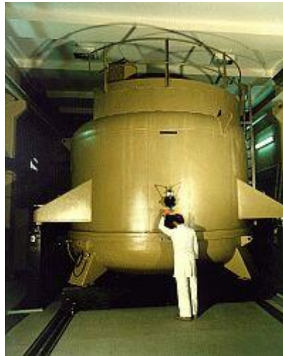
Fig. 2-41: aluminizing plant. Credit: ING
