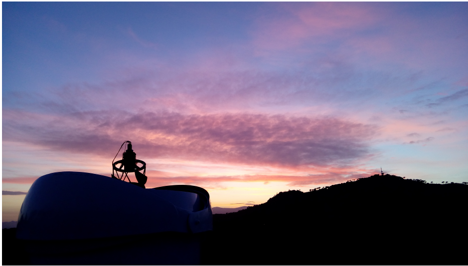
Figure 2.6: View of the Cebros TBT Observatory at sunset. All the telescope equipment, control and processing computers are hosted inside of the 4.2 m diameter clamshell dome.
