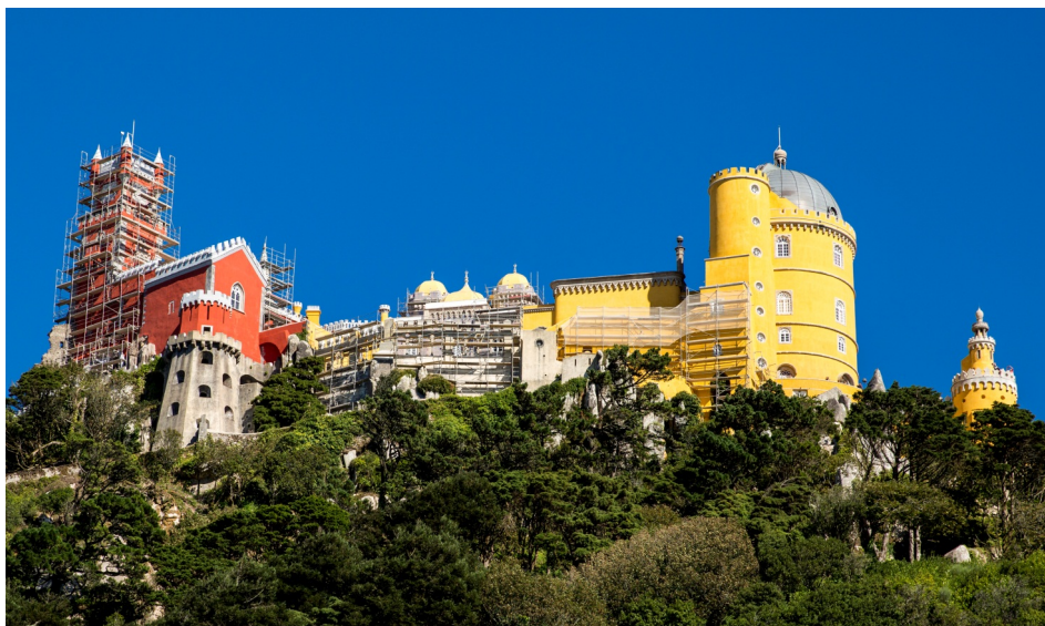
Figure 4 – Restoration of the facades, stone masonry and tiles
