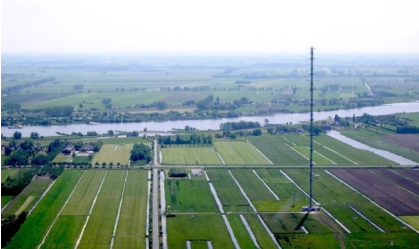
Figure 2.3: Aerial view of CESAR with the 200-m tower.
