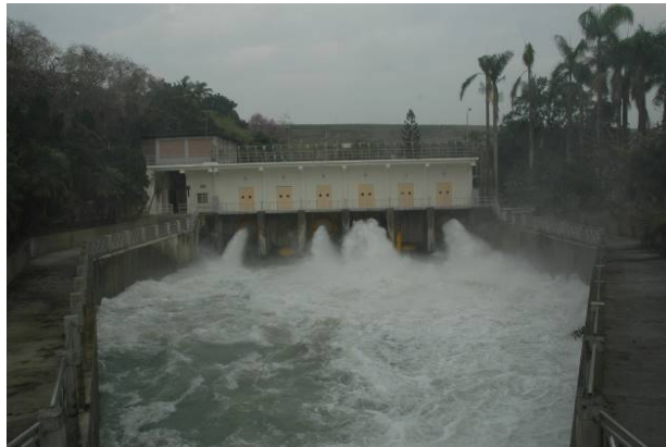
Figure 7: The facilities related to Jianan Irrigation System.
