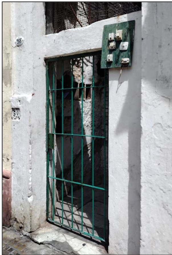
Figure 14 Several doorbells at the gate
