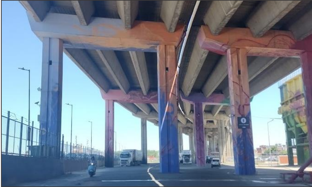
Figure 5 The road to La Boca
