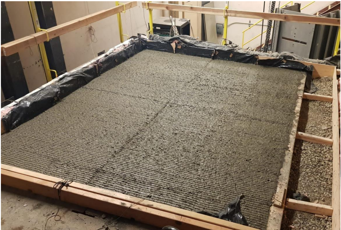
Figure 12. Immediately Tinned-Finished Concrete Slab.
