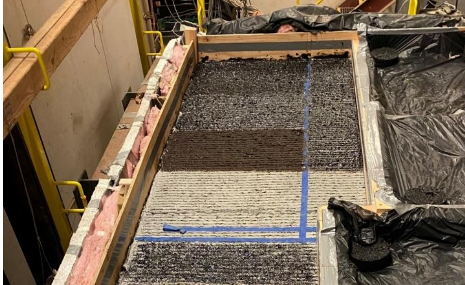
Figure 15. Uniform Tack Coat Application on New PCC Pavement Surface.
