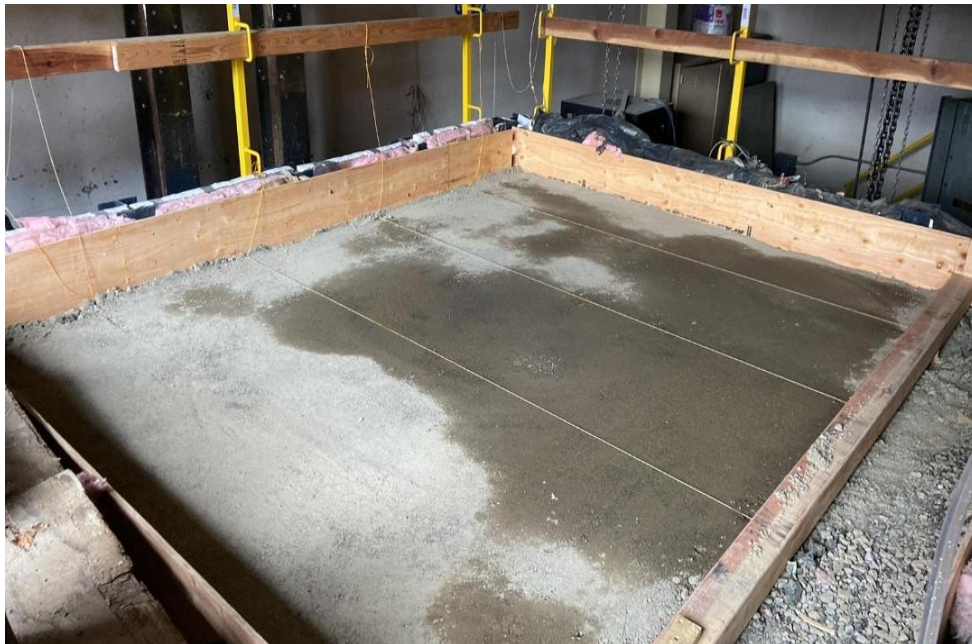
Figure 11. Aggregate Base Course Surface Leveling prior to Pouring PCC Slab.
