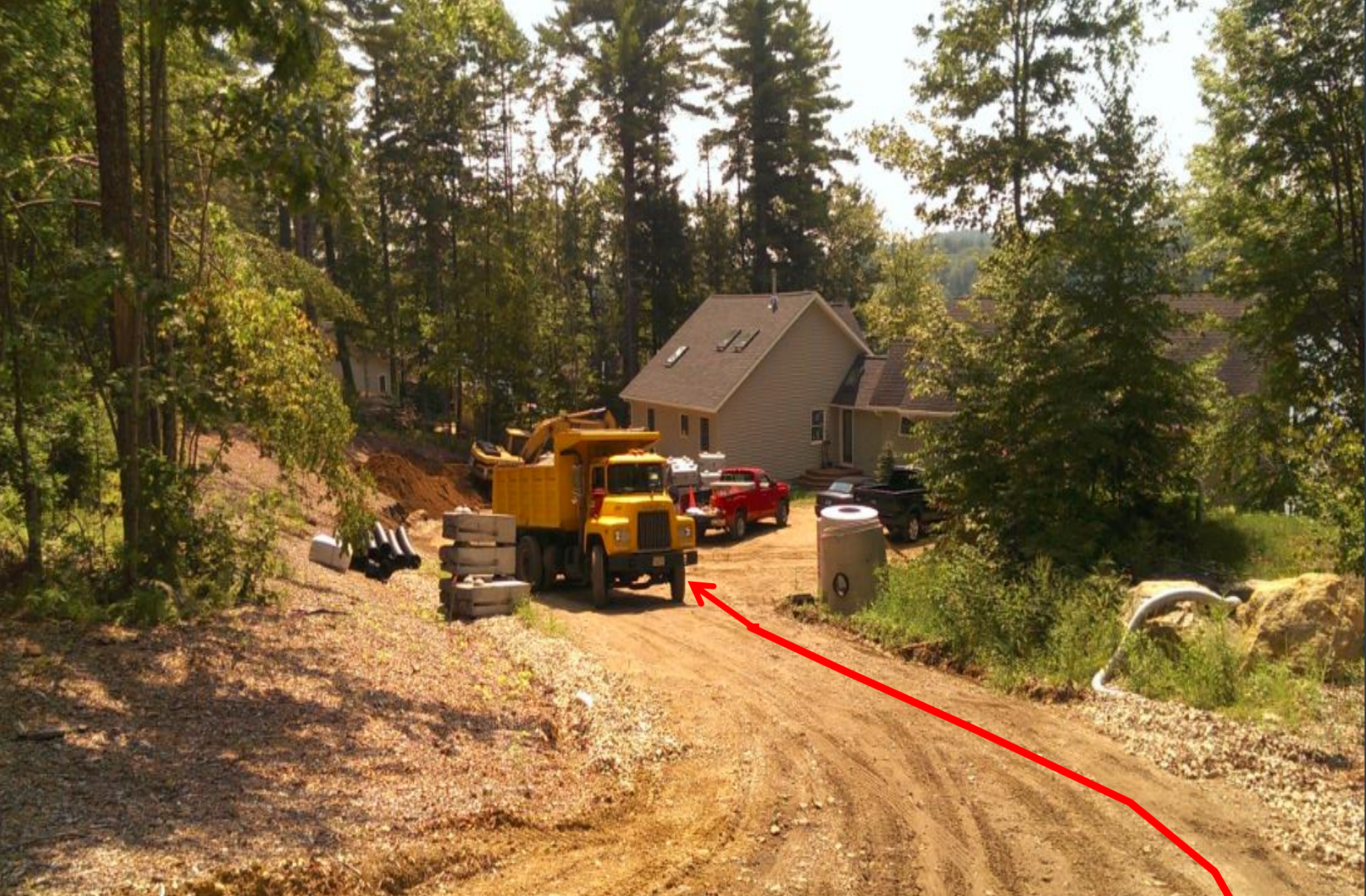
On this property, stormwater was directed to this detention area.
