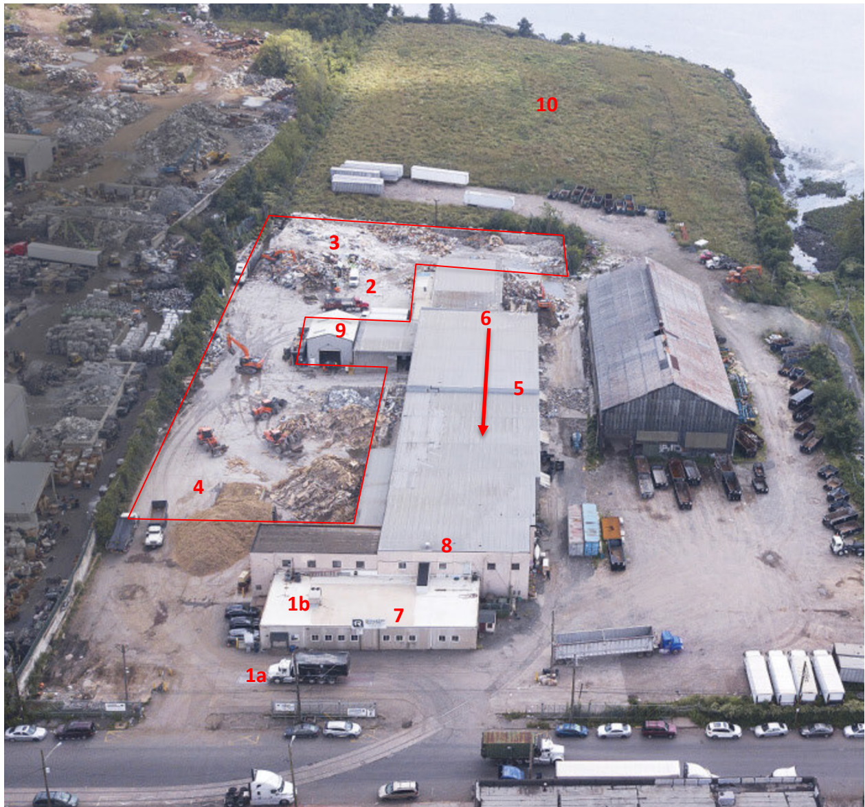
Figure 4. A drone photo of Revolution Recovery's Tacony facility, taken from the north; Milnor Street is in the foreground, and the Delaware River is in the background. Visible are a truck being weighed on the scale (1a) and measured in the scalehouse (1b), the tipping floor (2) within the broader yard (red outline), piles of partially sorted material (3) and sorted wood chips (4), the main building (5), the location of the sort line (inside the building; beginning around location 6 and moving towards Milnor Street), Billy's office (7), the studio (8, on second floor), the mechanical shop (9), and Metal Bank (10). Milnor Street is in the foreground, and the Delaware River is in the background. 8
