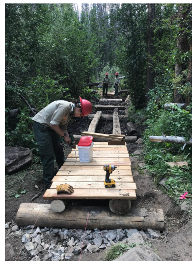
Figure 8. Installation of natural timber puncheon
