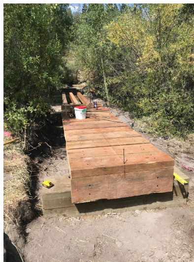
Figure 7. Installation of decking
