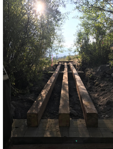
Figure 6. Stringers placed on mud sills
