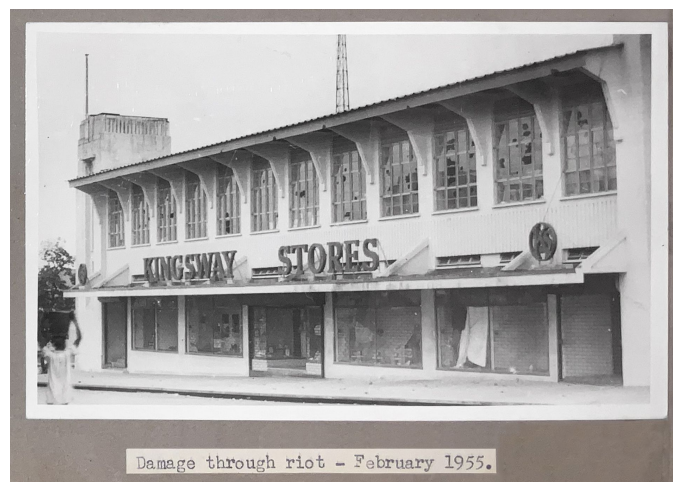
Photographer Unknown. Kingsway store Freetown, Sierra Leone. Damage through riot - February 1955. UAC/1/11/9/44/129 © Unilever Art, Archives and Record Management.
