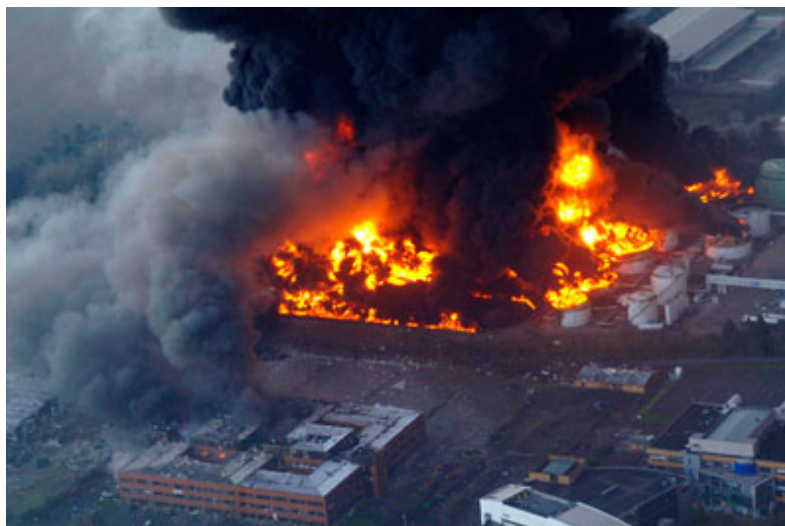
Figure 5.8 - Buncefield tank farm fire, which occurred on the 11th December, 2005, in Hertfordshire, England (48)
