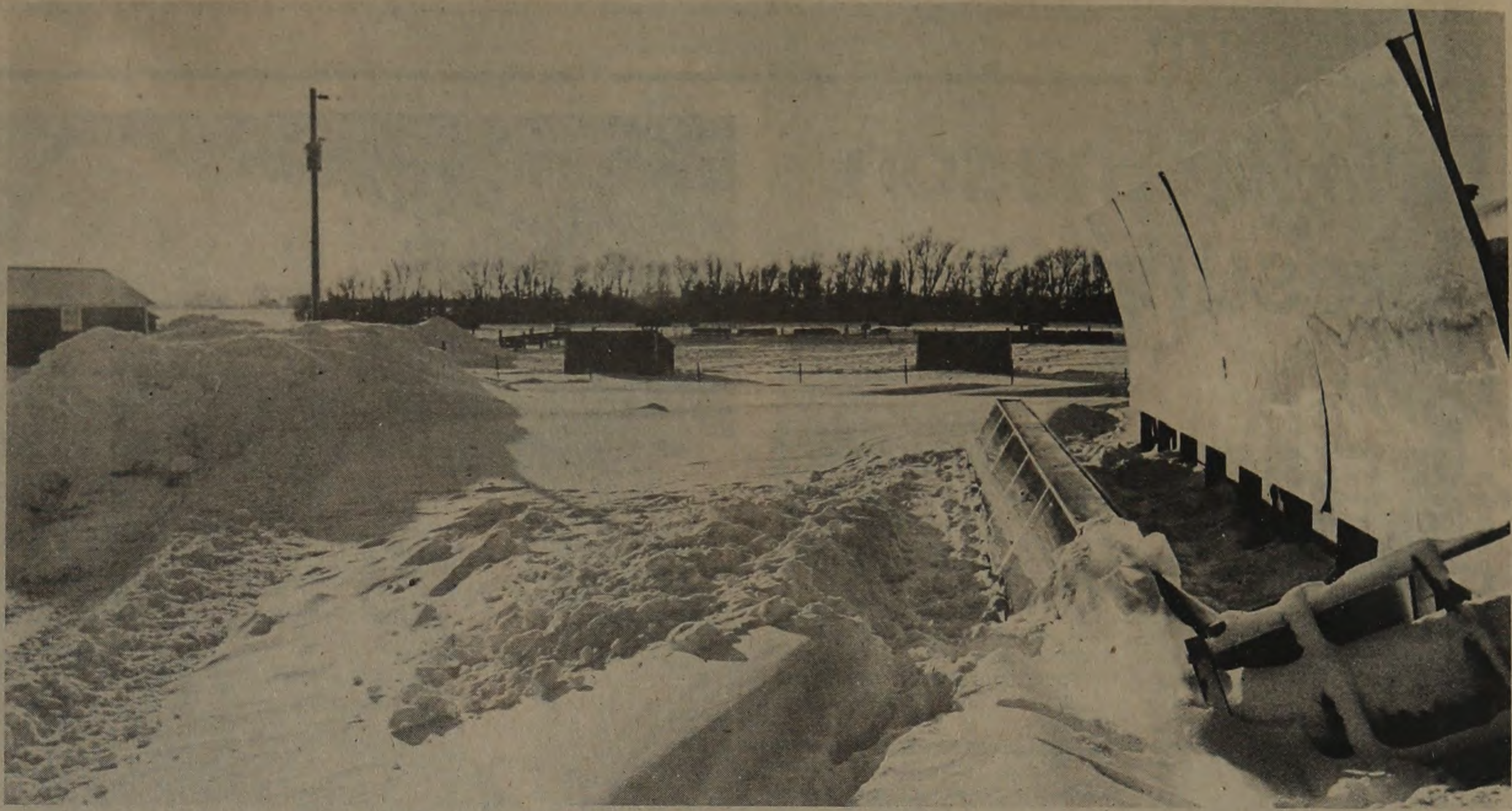
The crisp January sun shines on SDSU's solar heating unit north on Highway 14. Project leader Mylo Hellickson says the large, shiny reflector (right) focuses rays on the collector. Photo by Dave Elenkiwich
