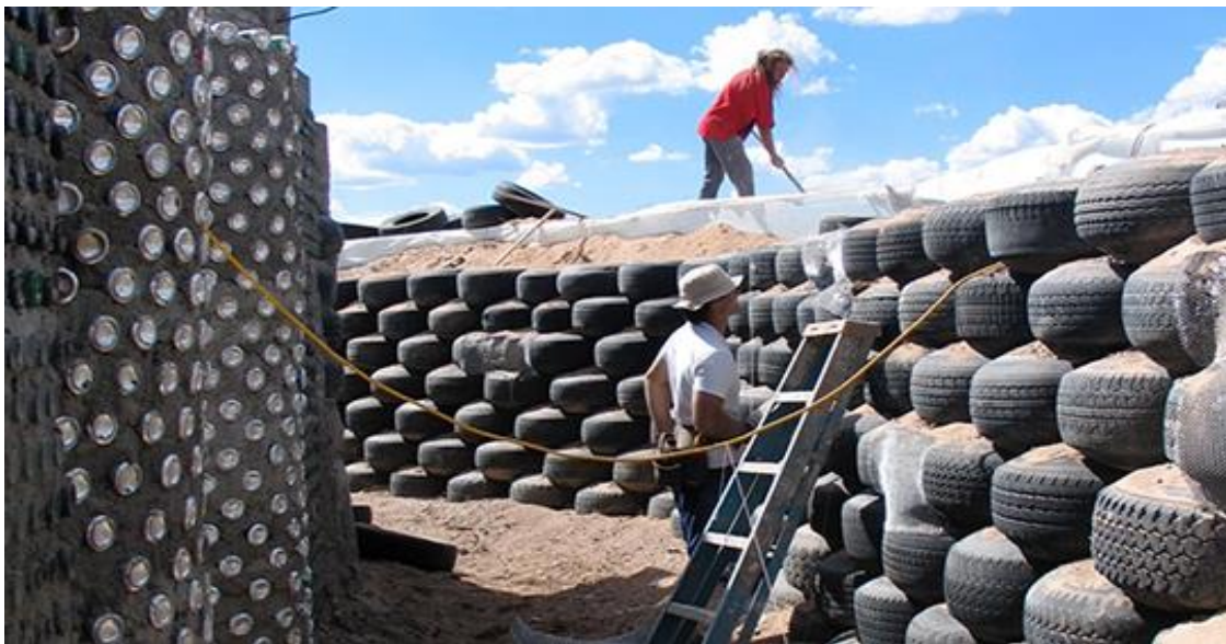
Figure 2: Tires Filled with Dirt in a Brick-Like Pattern (Earthship Bioteecture, 2023).
