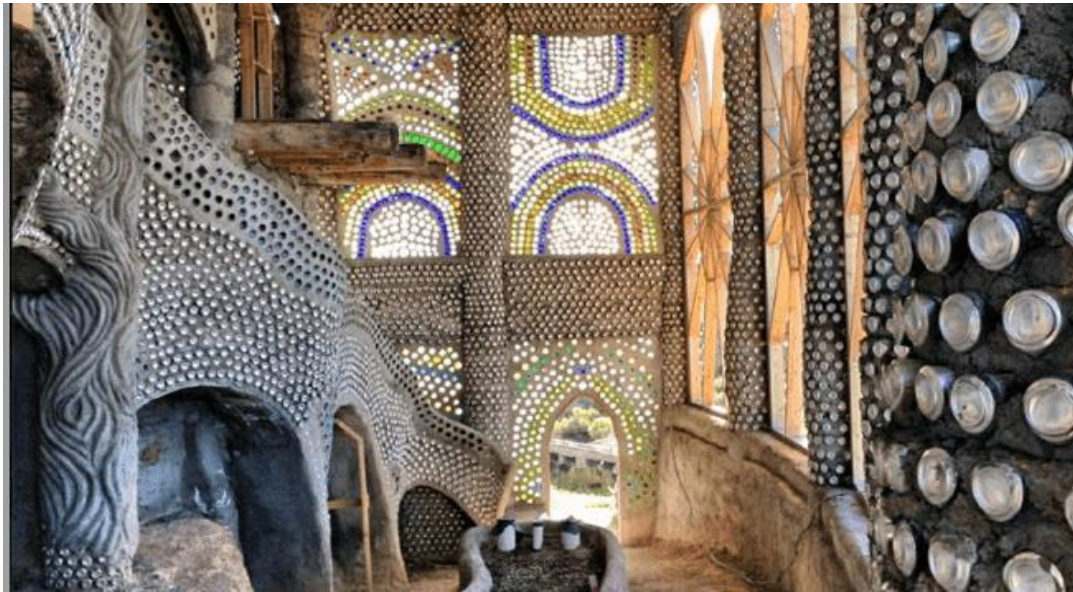
Figure 3: The Interior Design of an Earthship with Metal Cans and Glass Bottles (Ecowatch, 2023).
