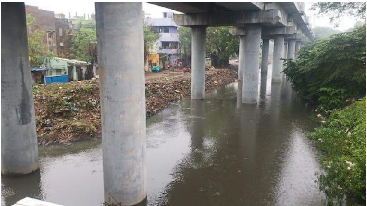
Figure 16. Buckingham Canal, partly dredged taking the floodwaters (Mylapore time, 2021)
