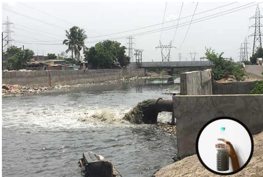
Figure 19. Untreated sewage pumped into Buckingham Canal (CMWSSB)
