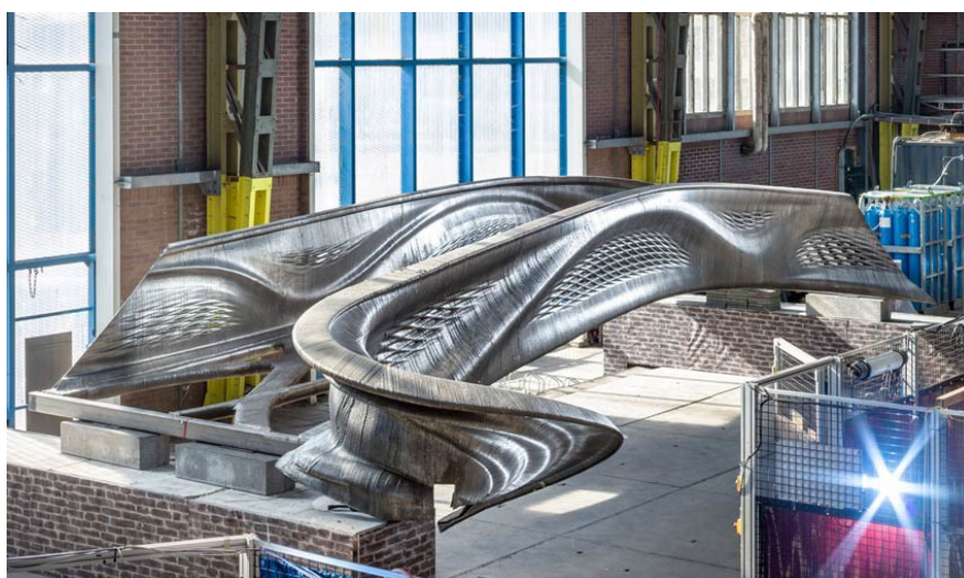
Figure 1.5: The world's first metal 3D printed steel bridge ( https://www.3dnatives.com/ )
