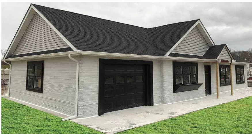
Figure 1.4: Concrete 3D printed home, New York ( https://www.inputmag.com/tech )
