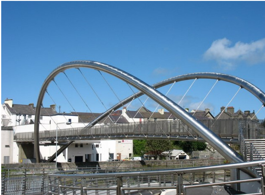
Figure 1.2: Stainless steel arch in the Celtic Gateway Bridge, UK ( https://structurae.net/en/structures/the-celtic-gateway-bridge )
