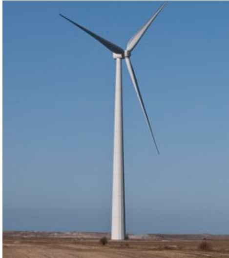
(a) Wind turbine tower
