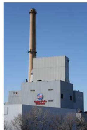
Image 2.1 Cedar Falls Utilities power plant.
